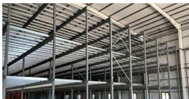
Bare steel mezzanine awaiting installation of decking and fire rating
